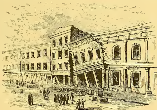
EARTHQUAKE SCENE IN SAN FRANCISCO.
